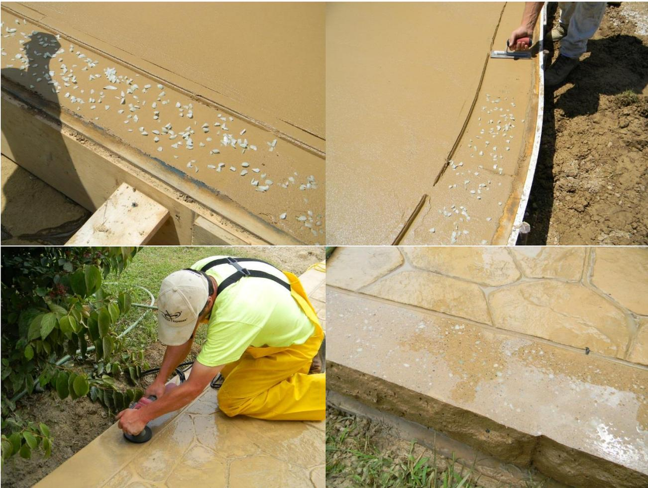
Top Left: Place Core Glow Commercial Grade Marble (Natural Stones) along project surface area once allotted time has passed. Surface should be stiff but not hard. Top Right: Press stones into the cement surface. Bottom Left: Sand down surface area once cement has set. Bottom Right: Finished concrete surface with glow stones embedded permanently in the surface.
